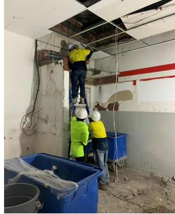
Demolishing of existing toilets, removal of Asbestos and construction of new disabled toilets in accordance with (DDA) 1992
