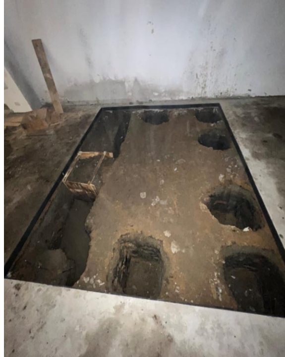
Demolishing of existing tenancy and preparation for the installation of a new 10.5 tone vault in accordance with National Construction Code (NCC) 2022.
