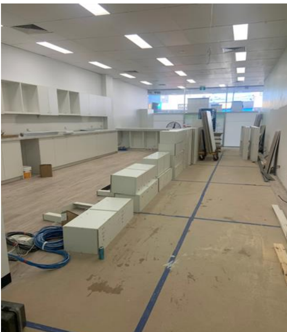
Construction of acoustically rated solid plaster walls, new air-conditioning system and installation of joinery in accordance with the Pharmacy Board
