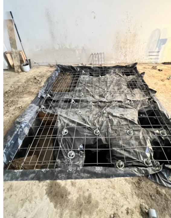
Demolishing of existing tenancy and preparation for the installation of a new 10.5 tone vault in accordance with National Construction Code (NCC) 2022.
