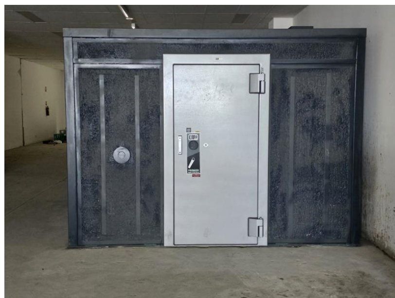
Construction of a new 10.5 tone vault to dispense Medicinal Cannabis in accordance with the Office of Drug Control (ODC) and the Pharmacy Board of Australia.
