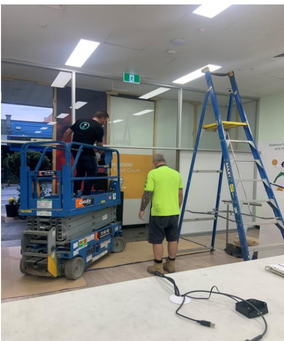
Removal of existing non-complaint shopfront and installation of new in accordance with National Construction Code (NCC) 2022
