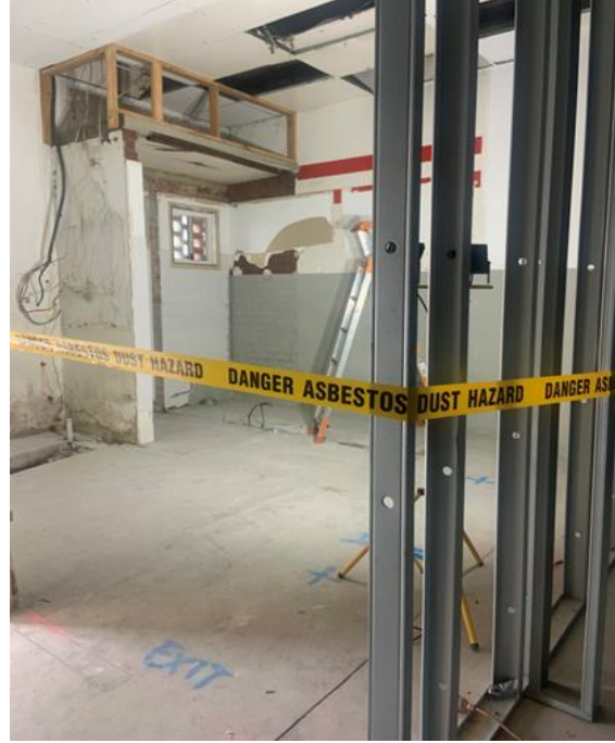
Demolishing of existing toilets, removal of Asbestos and construction of new disabled toilets in accordance with (DDA) 1992
