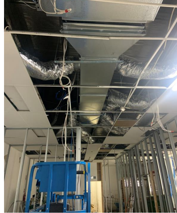
Construction of acoustically rated solid plaster walls, new air-conditioning system and installation of joinery in accordance with the Pharmacy Board
