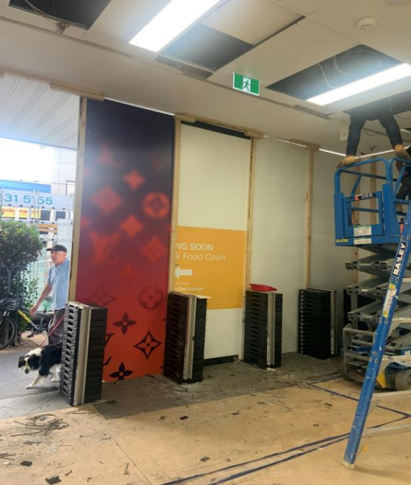
Removal of existing non-complaint shopfront and installation of new in accordance with National Construction Code (NCC) 2022
