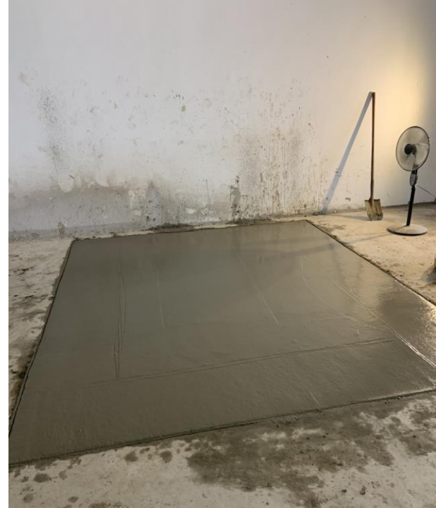
Demolishing of existing tenancy and preparation for the installation of a new 10.5 tone vault in accordance with National Construction Code (NCC) 2022.
