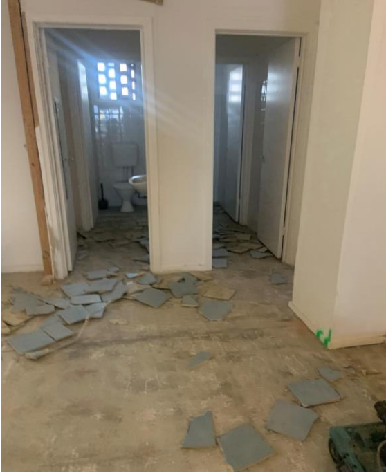
Demolishing of existing toilets, removal of Asbestos and construction of new disabled toilets in accordance with (DDA) 1992
