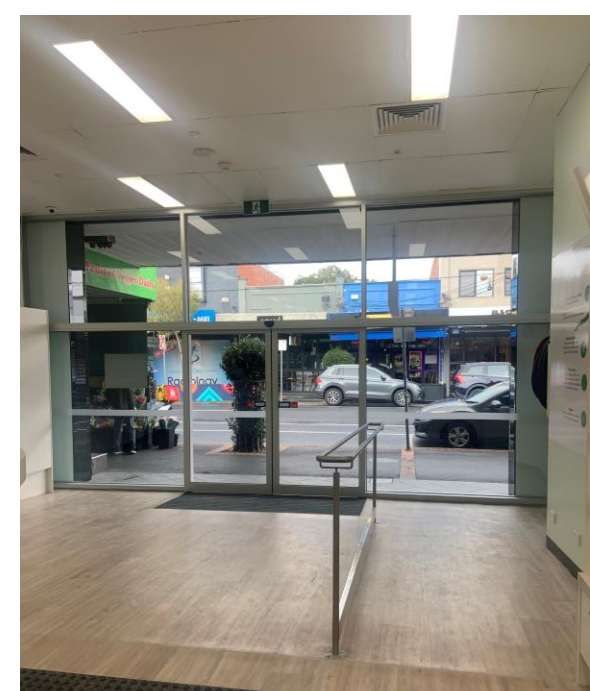
Removal of existing non-complaint shopfront and installation of new in accordance with National Construction Code (NCC) 2022
