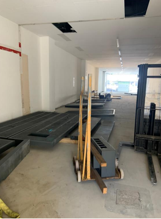
Construction of a new 10.5 tone vault to dispense Medicinal Cannabis in accordance with the Office of Drug Control (ODC) and the Pharmacy Board of Australia.
