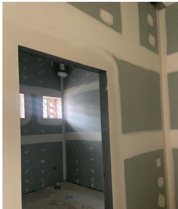
Demolishing of existing toilets, removal of Asbestos and construction of new disabled toilets in accordance with (DDA) 1992
