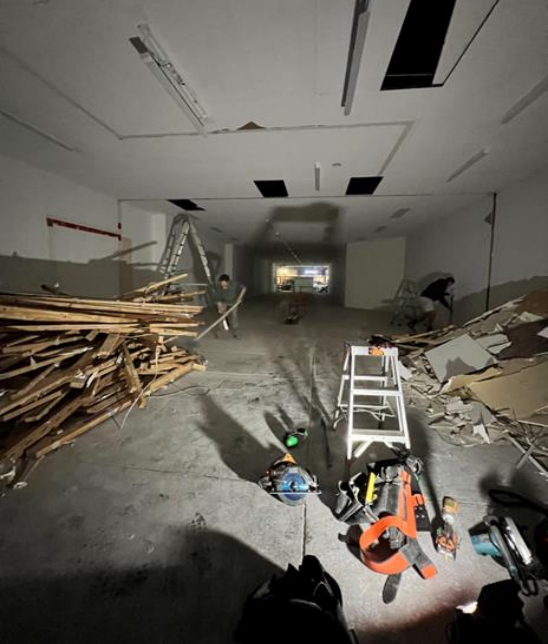
Demolishing of existing tenancy and preparation for the installation of a new 10.5 tone vault in accordance with National Construction Code (NCC) 2022.
