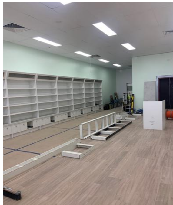
Construction of acoustically rated solid plaster walls, new air-conditioning system and installation of joinery in accordance with the Pharmacy Board
