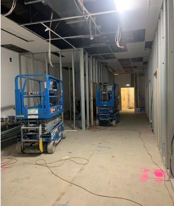
Construction of acoustically rated solid plaster walls, new air-conditioning system and installation of joinery in accordance with the Pharmacy Board
