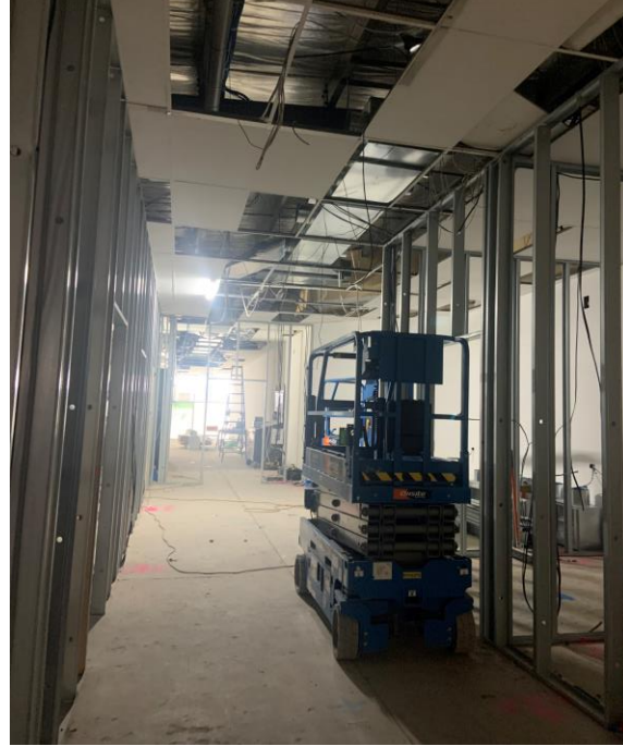
Construction of acoustically rated solid plaster walls, new air-conditioning system and installation of joinery in accordance with the Pharmacy Board
