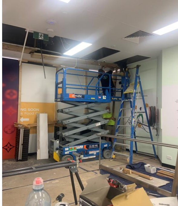
Removal of existing non-complaint shopfront and installation of new in accordance with National Construction Code (NCC) 2022
